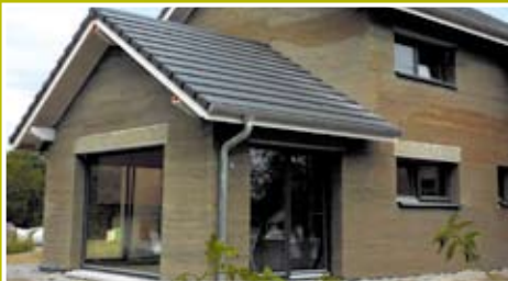
INSULATION OF WALLS
