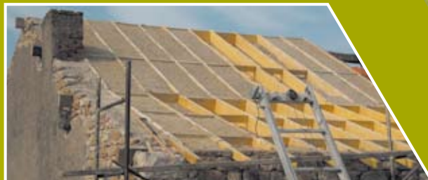
INSULATION OF ROOFS
